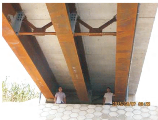
Fig. 21 Cross section of main girder
